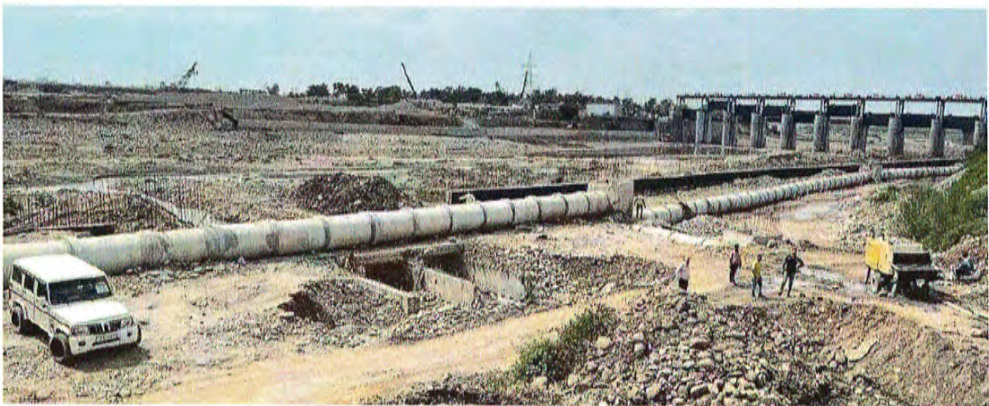
Picture showing Interceptor Drain On Left Bank
