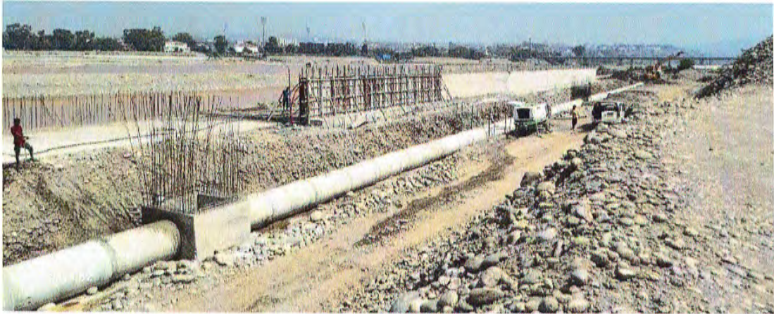
Picture showing Interceptor Drain On Left Bank
